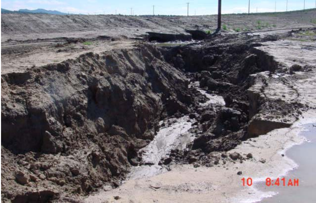
Severe erosion from a precipitation event caused by inadequate sediment and erosion controls.
