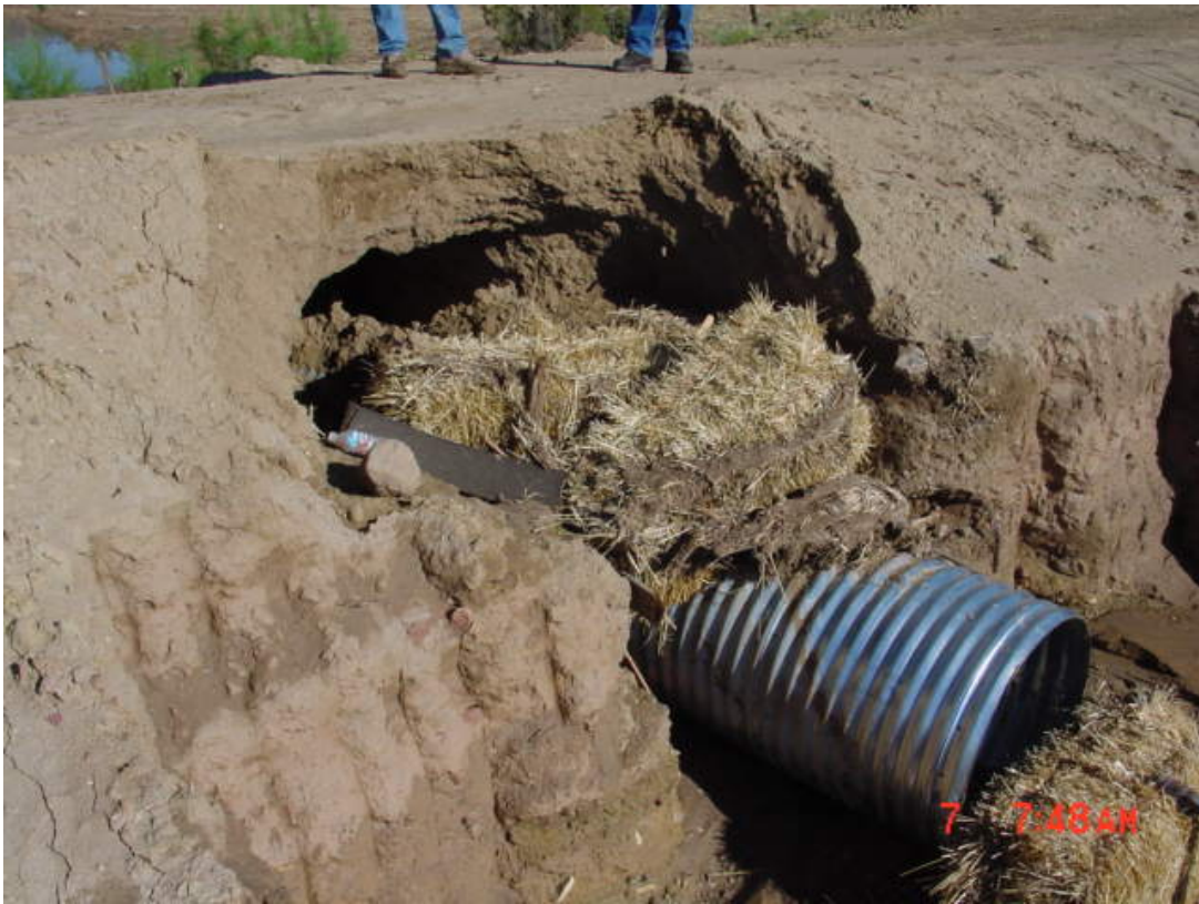
Improper installation of sediment and erosion controls caused a failure in the drainage system in a new sub-division
