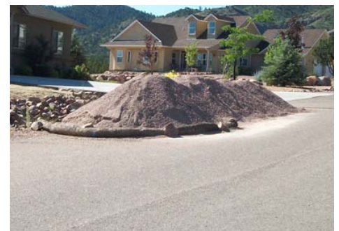
BMP in place
