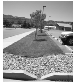
Rain gardens fed by passive rainwater harvesting border the buildings and parking lots of the TAD redevelopment project in Denver, CO. The rain gardens beautify the site, reduce the urban heat island effect, and provide habitat, while reducing runoff to the nearby South Platte River. Photo courtesy of Brook Associates.
