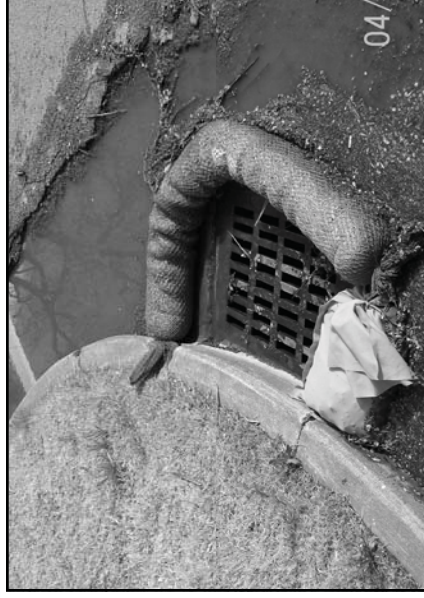
Properly installed inlet protection keeps sediment and other debris from discharging into the stormdrain & ultimately into the Arkansas River
