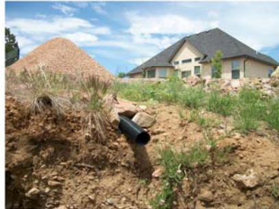
Roof Drain; Once marked doesn't need inspected unless a problem is noted.
