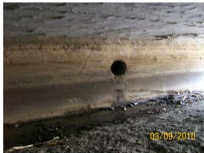
Field connection to inside of bridge or culvert. Always mark and record.
