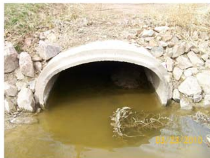
Elliptical RCP Measure both Horizontal and vertical diameters
