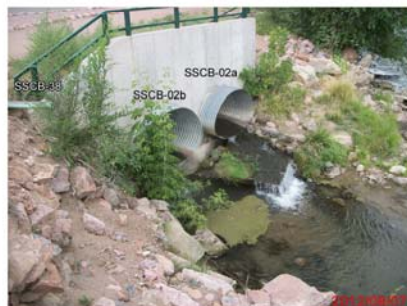
Double Outfall; Mark as separate outfalls unless known to have the same origin.
