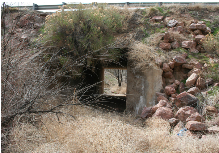
Existing Box Culvert At Hwy 115
