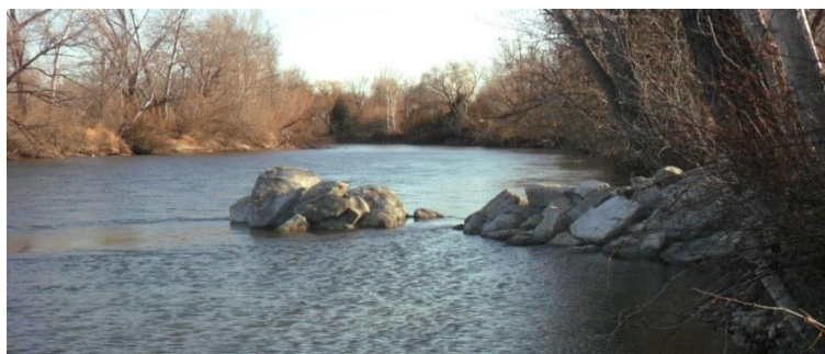
Jetties can be placed along the river's edge to create eddies, stabilize river banks, and create interesting currents for river recreationalists. These should be considered throughout this entire reach. However due to flood conveyance and river stabilization issues, detailed modeling and evaluation are needed to determine placement and design. This is well beyond the scope of this effort and should be included in future planning efforts.
