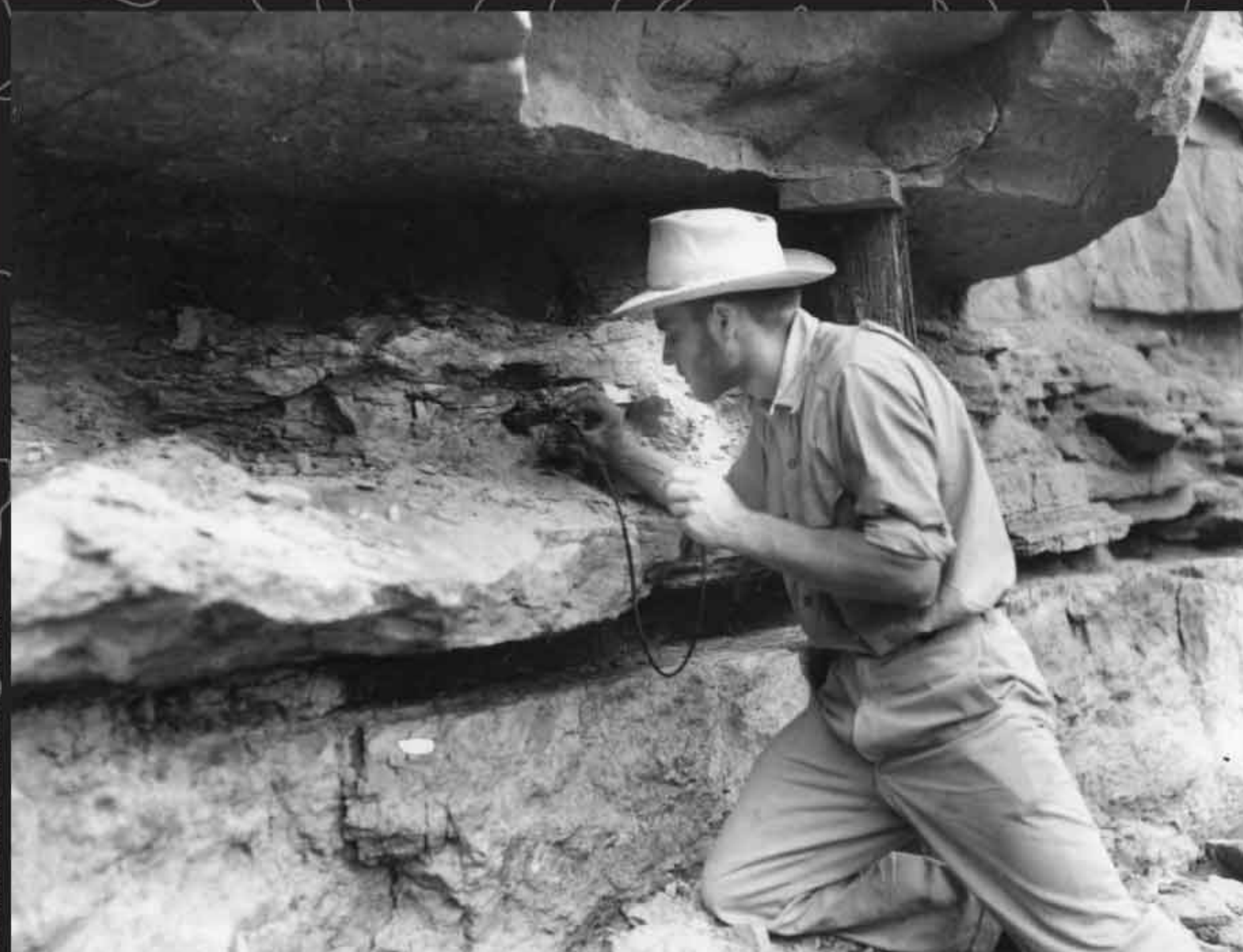
Edwin Delfs setting a charge beneath an unstable rock shelf
