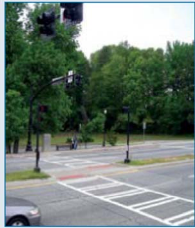
Figure 7. PHB installed on Buford Highway near pedestrian attractors: a transit stop.
